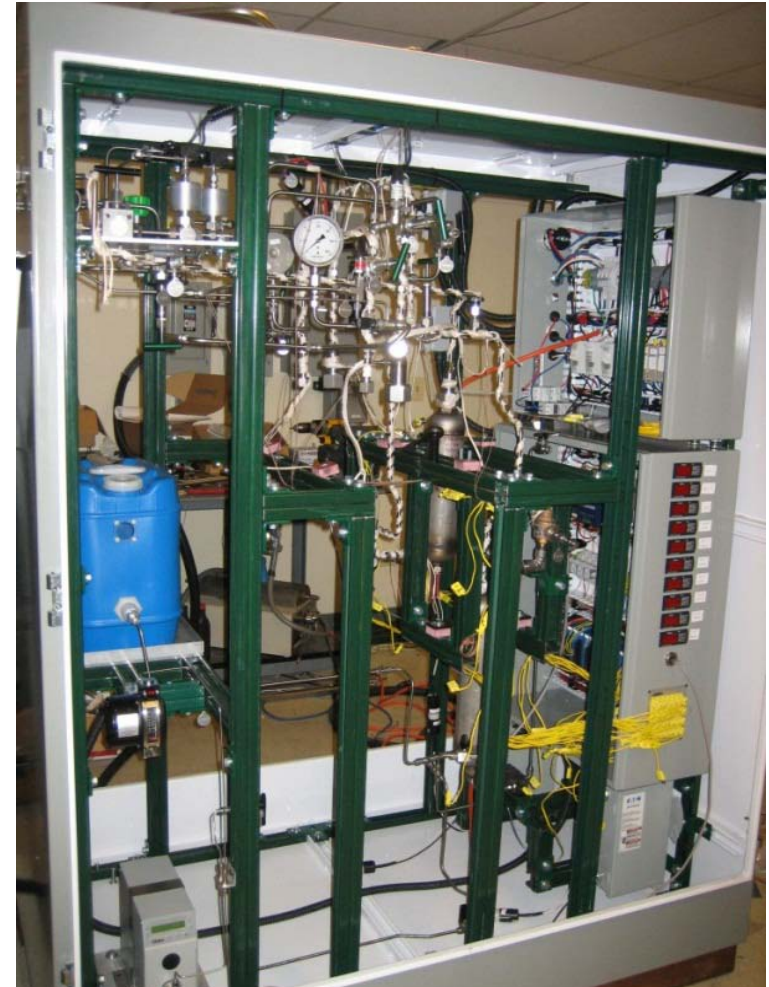
Gas Conditioning Skid
