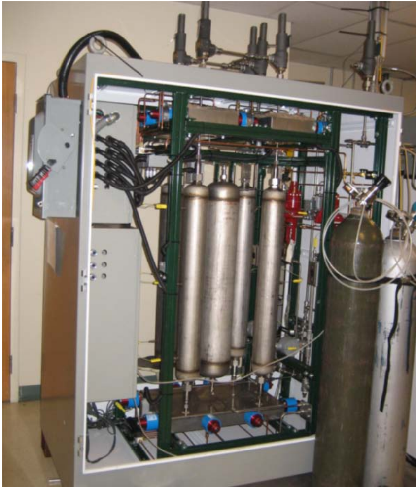
CO 2 Removal Skid
