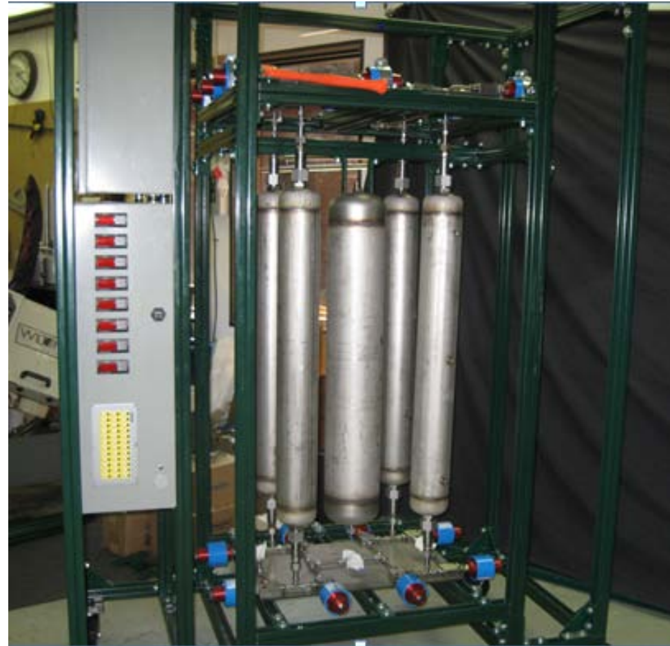
Skid #2 - CO 2 removal skid
